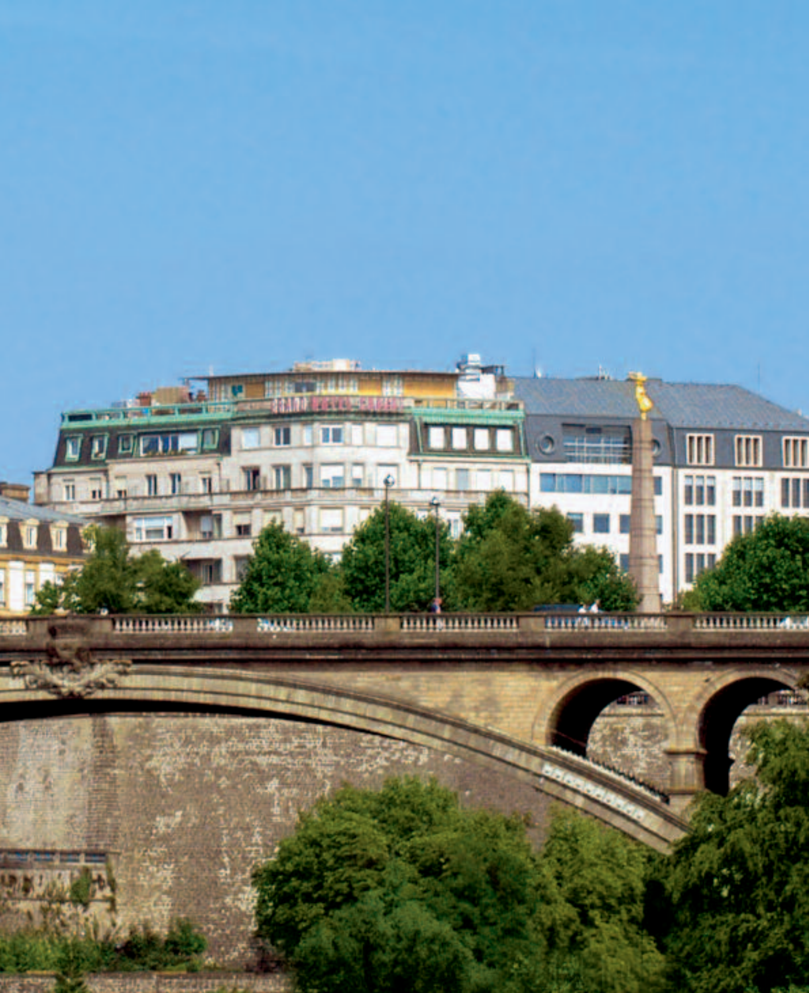
LUXEMBOURG Adolphe Bridge
